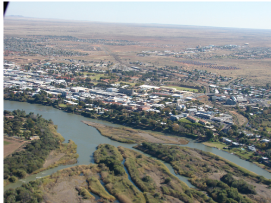
Aerial view of Upington
